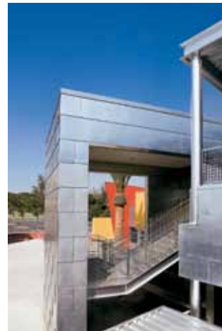
Galvanized metal stairwell
